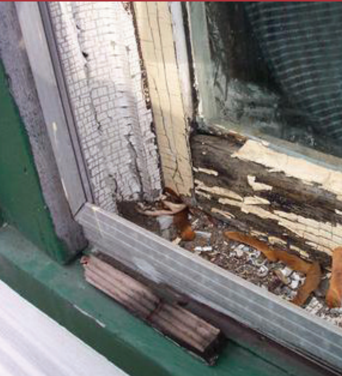
Window with chipping and peeling lead-based paint
