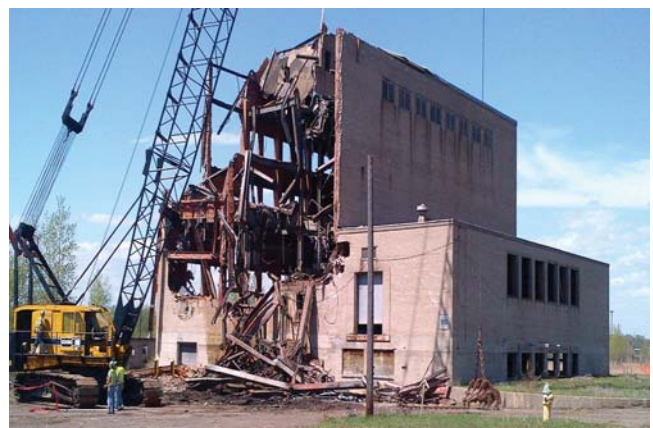
Crews demolish one of the remaining buildings at the former Twin Cities Army Ammunition Plant. Now named Rice Creek Commons, the 427-acre development will include a mix of residential, commercial and open spaces.
