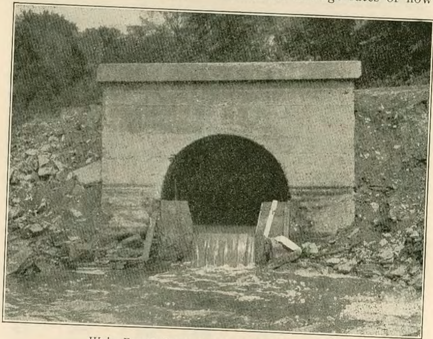
Weir, Fourth Street South, Outlet, Minneapolis Average discharge, 1,570,000 gallons per 24 hours
