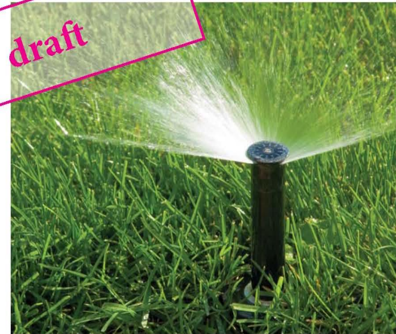
Irrigation re-use of treated stormwater in demonstration area within district
