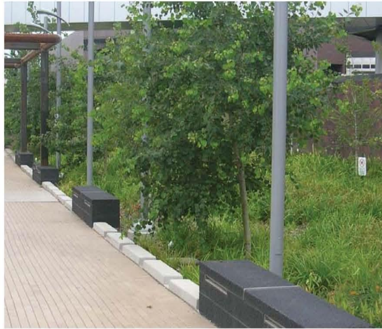
Large-scale raingardens that filter and evapo-transpirate untreated water – 3:1 slopes, 2' deep
