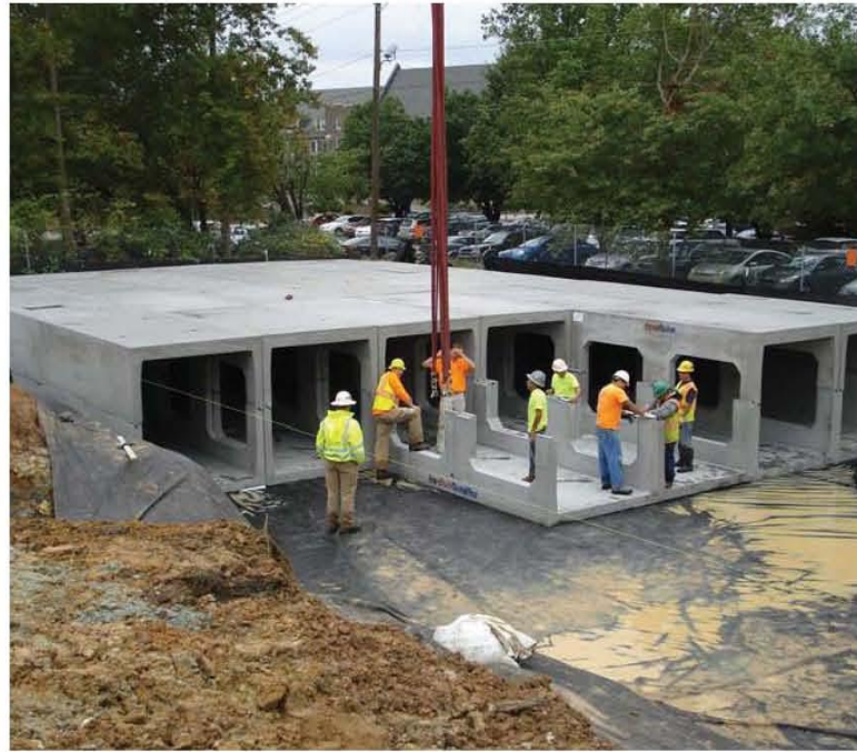
Underground storage cells for treated stormwater retention – 6x8' cells, buried under park area
