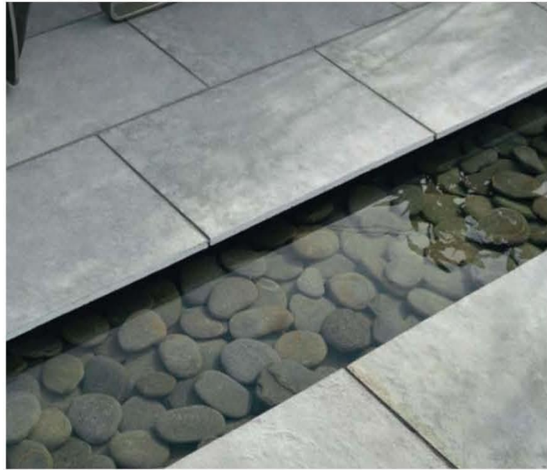
Ornamental surface gutters for untreated stormwater – roof water and surface runoff
