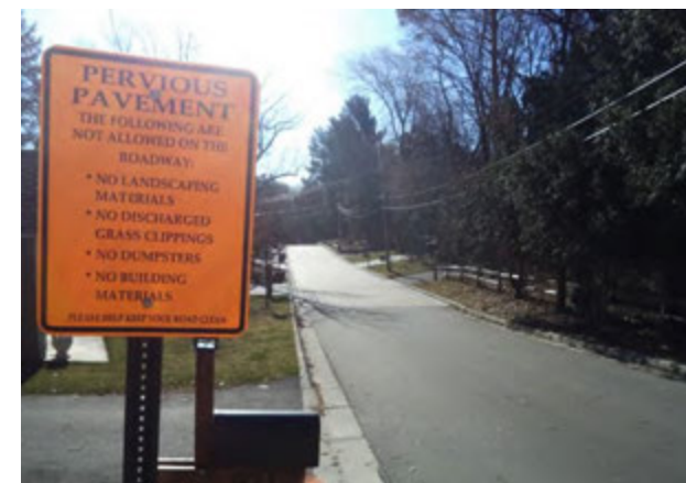
Pervious Pavement, photo by Ashley Bennett
