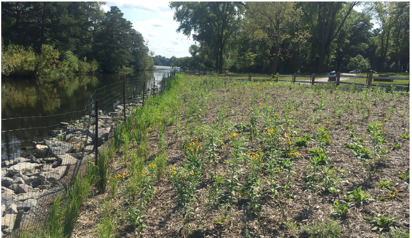
Completed Sucker Lake Channel Restoration with native planting
