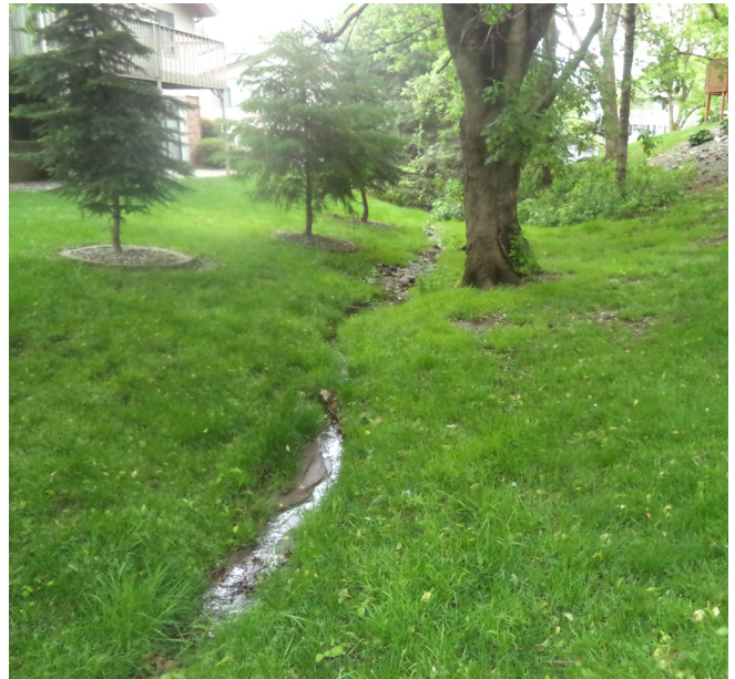
Rolling Hills raingarden original eroding condition
