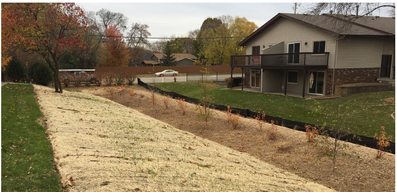
Completed Rolling Hills Raingarden. Project collects, infiltrates, and filters stormwater from the HOA property.
