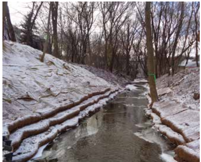
Stabilized condition of the Phase 4 reach of Lambert Creek. Planting to be installed in spring 2017.
