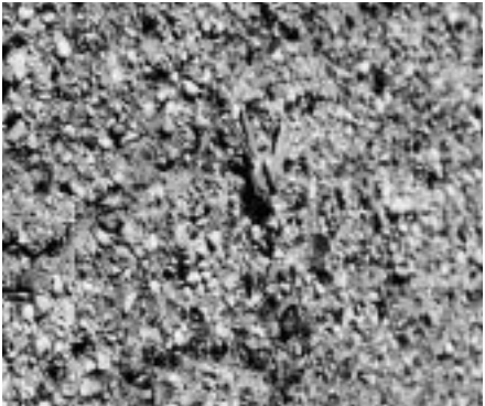
Severe ravelling with ▼ extreme loss of aggregate.
