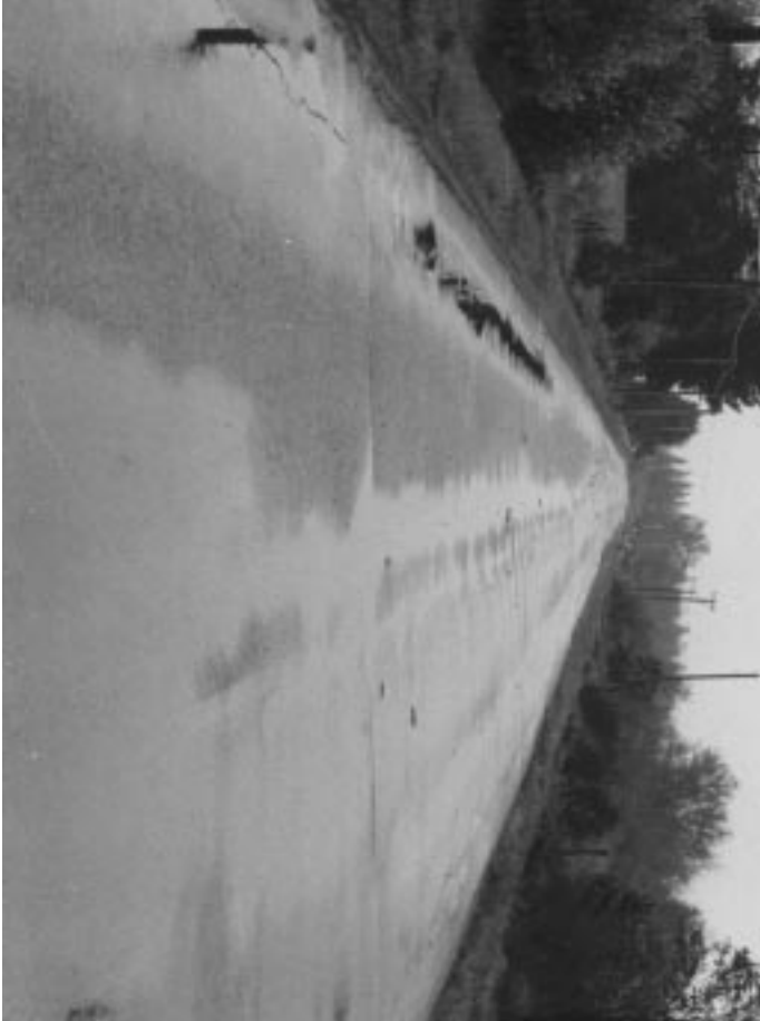
▶ Even slight rutting is evident after a rain.
