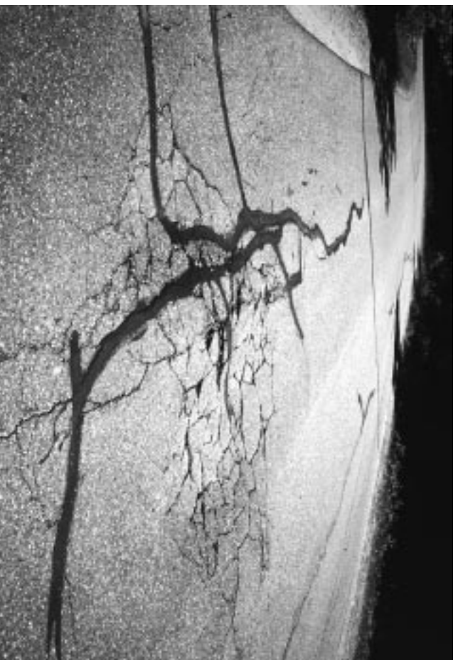
▶ Frost heave damage from spring break-up.
