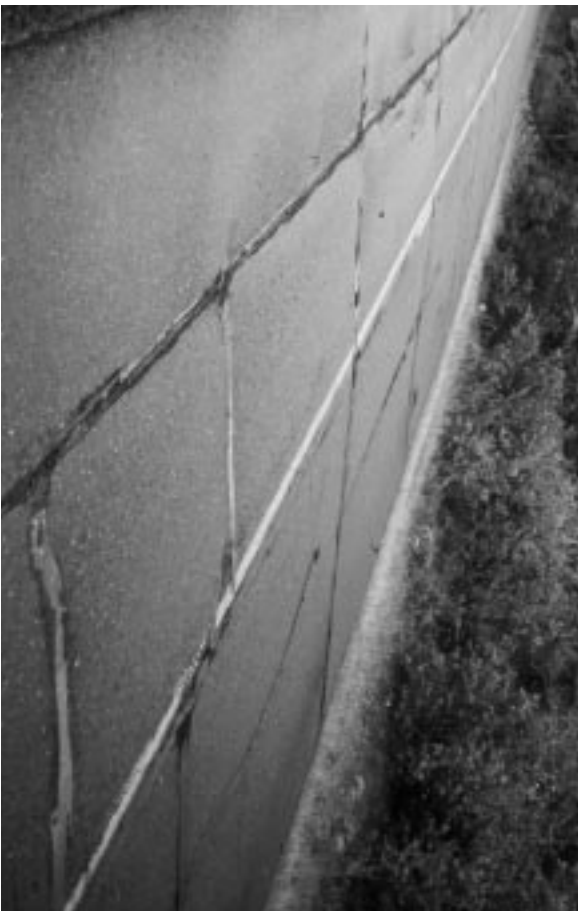
▶ Concrete joints reflected through bituminous overlay.
