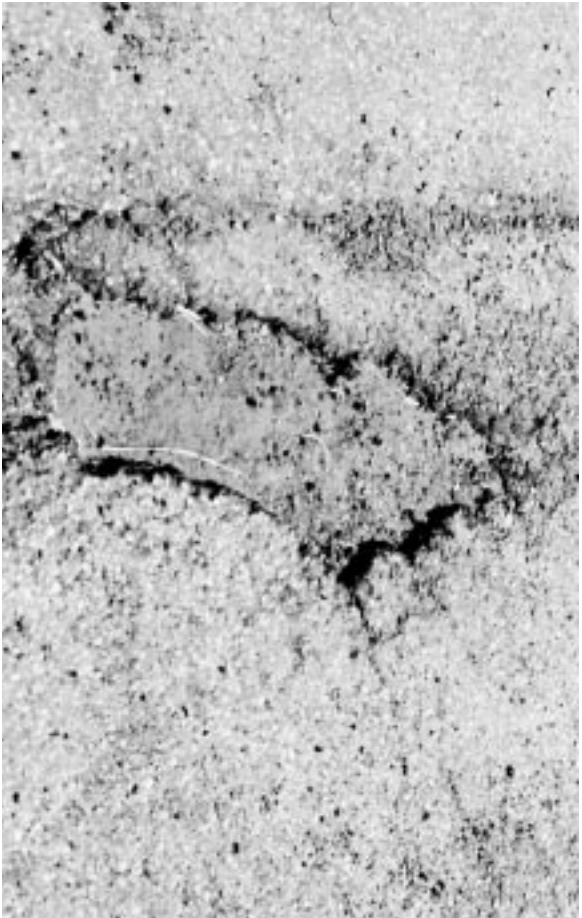
▶ Small pothole where top course has broken away.
