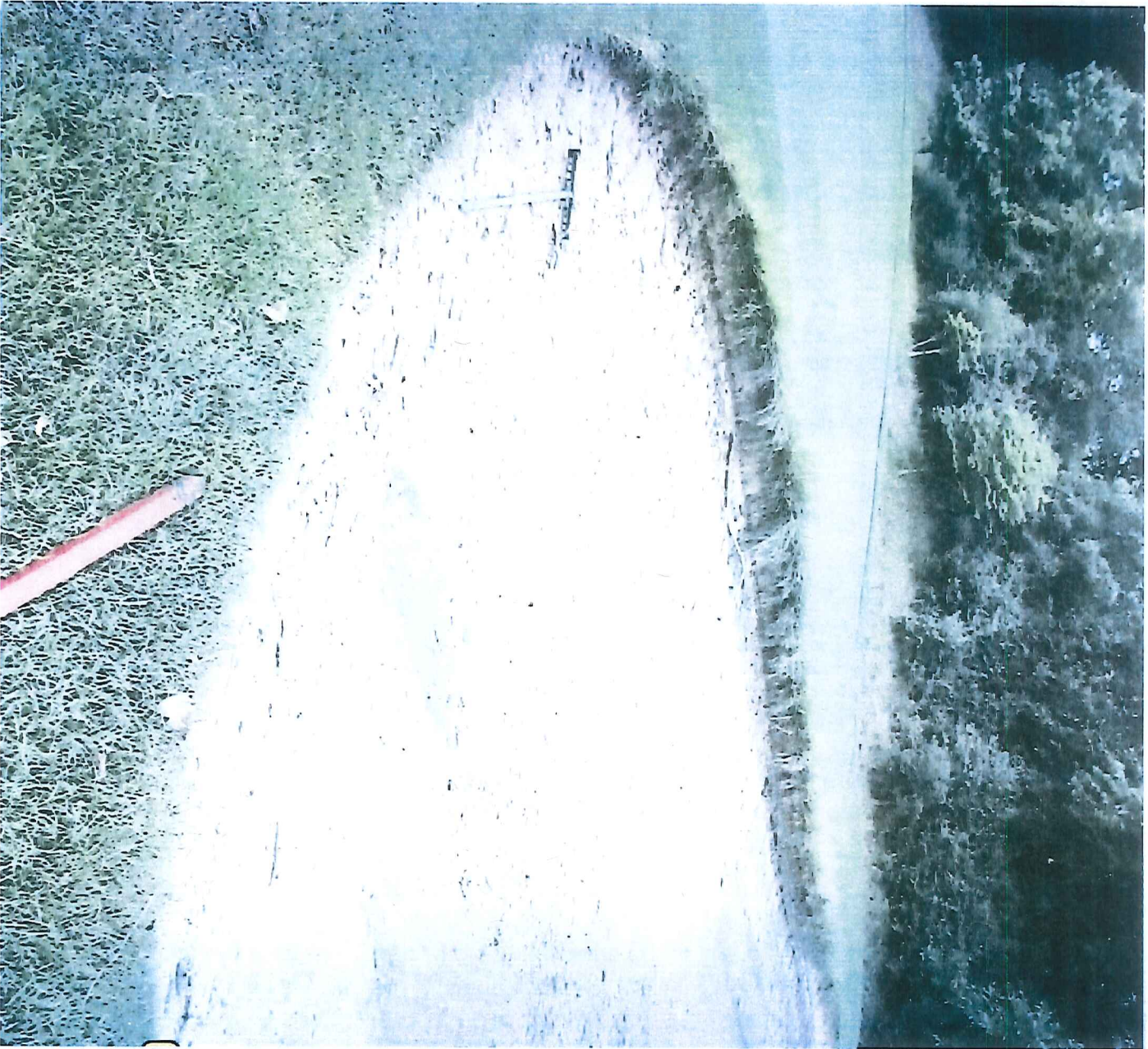
An example of a contaminated bunker as a result of drainage failure
