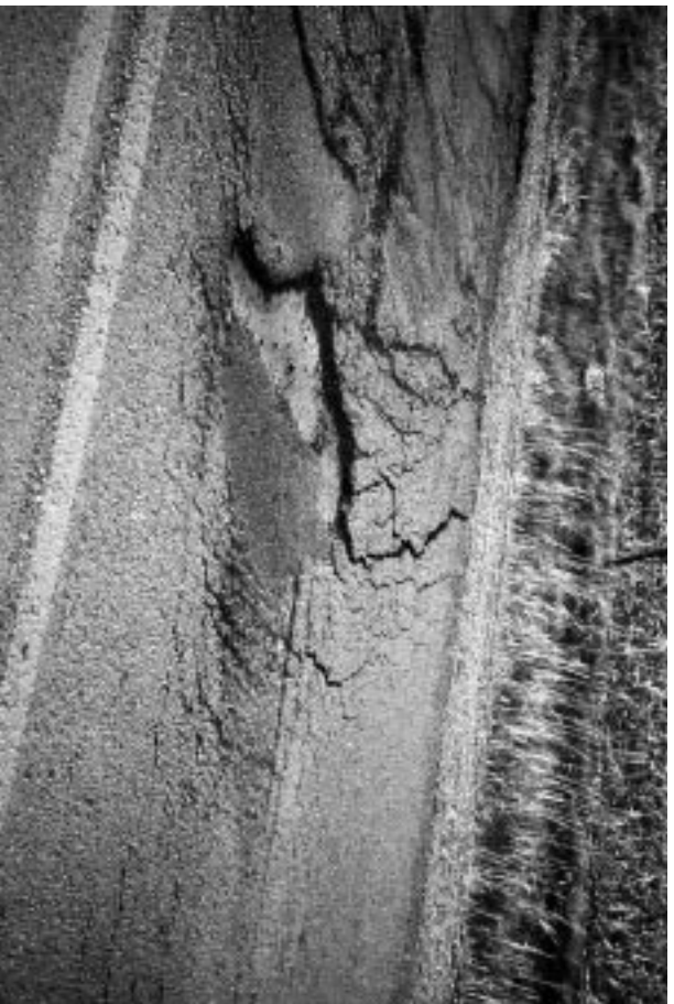
▶ Loss of bond between pavement layers allows traffic to break loose pieces of surface.
