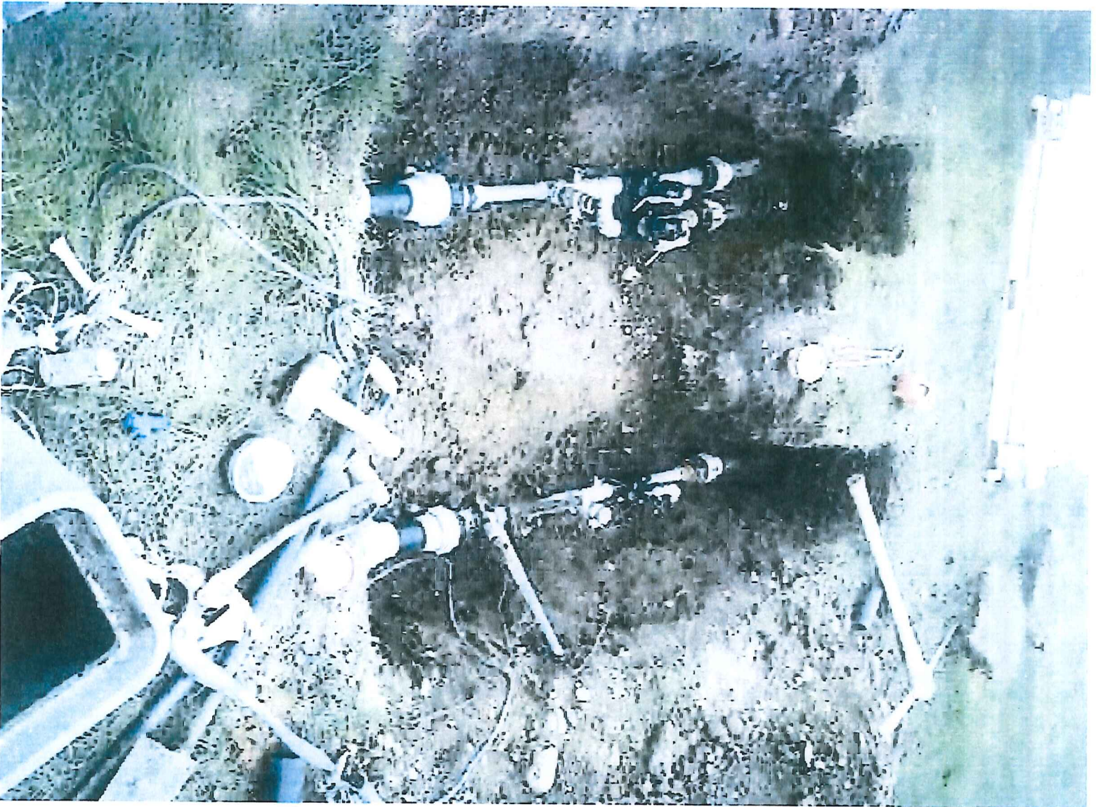
Example of turf disruption for repairs to irrigation system.
