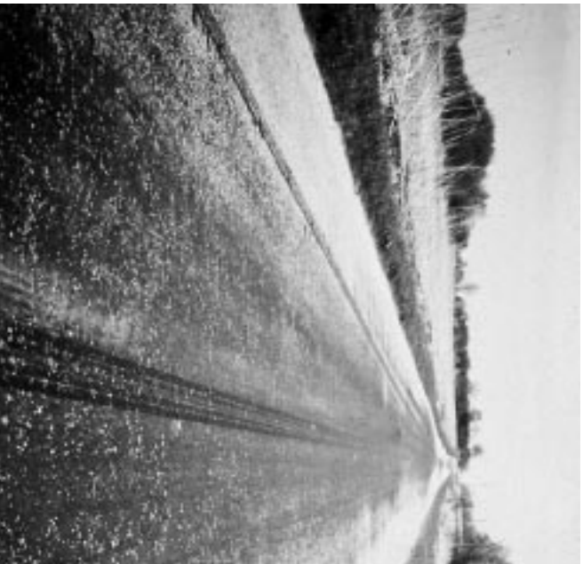
▼ Wedges and patches extensive but in good condition.
