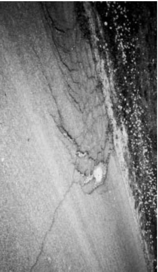
▶ Crescent-shaped cracks characteristic of slippage.
