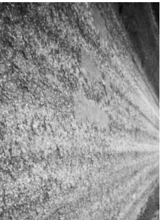
▶ Severe raveling and loss of surface material.
