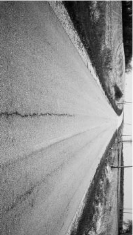
▼ Slight rutting; patch in good condition.
