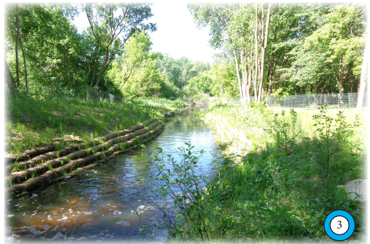
LAMBERT CREEK- Native planting and shoreline stabilization
