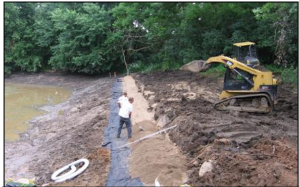
2011 Clean Water Funds were used to help the Capitol Region Watershed District make a pond improvement, which included an iron enhanced sand filter.
