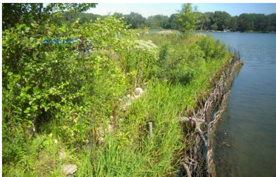
Shoreline restoration project on Lake McCarron's
