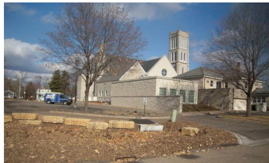
Bioinfiltration basin within VLA WMO installed to collect runoff from St. Mary's Church and Parking Lot
