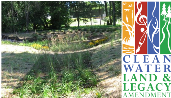
Bioinfiltration basin installed along Aladdin Street in Roseville, MN with funding provided by the Clean Water Land & Legacy
