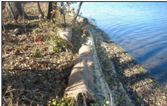
2011 BWSR Cost-share Funding was used to restore Lake Johanna shoreline.
